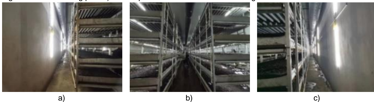
Fig. 6 - Interior environment of mushroom house
