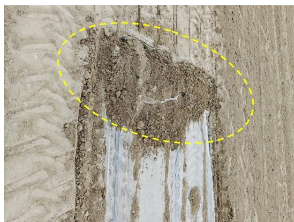
(b) Effectiveness of landfill liner installation
