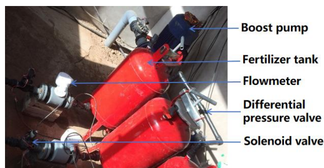
Fig. 1 - Primary equipment configuration plan
