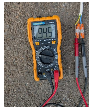
Fig. 16 - Measuring the output voltage
