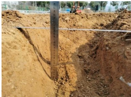
Fig.14 - Process of Measuring Trench Depth
