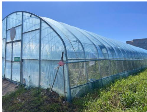
Fig. 1 – Flat-elliptical pipe greenhouse
