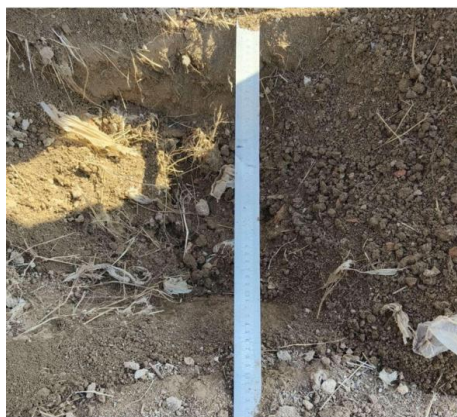
Fig. 11 – Trenching width measurement
