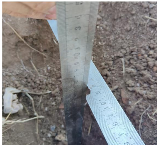
Fig. 10 – Trenching depth measurement
