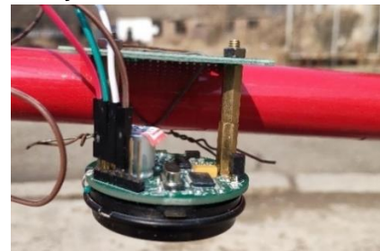
(b) Installation Position of KS109
