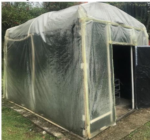
Fig. 3 - Double-layer polyethylene marquee used
