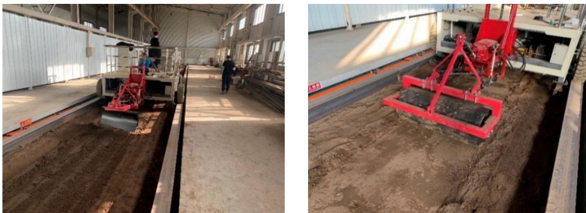
Fig. 4 - Picture of soil preparation
