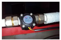
Fig. 8 – Installation of volumetric flow meter to the panel (DV1)
