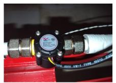
Fig. 9 - Installation of volumetric flow meter to the gasifier (DV2)
