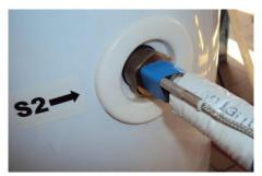
Fig. 6 - Installation of thermal detector to the boiler outlet (S3)
