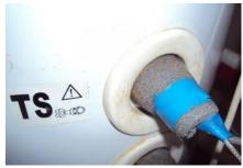
Fig. 5 - Installation of thermal detector to the boiler inlet (S2)
