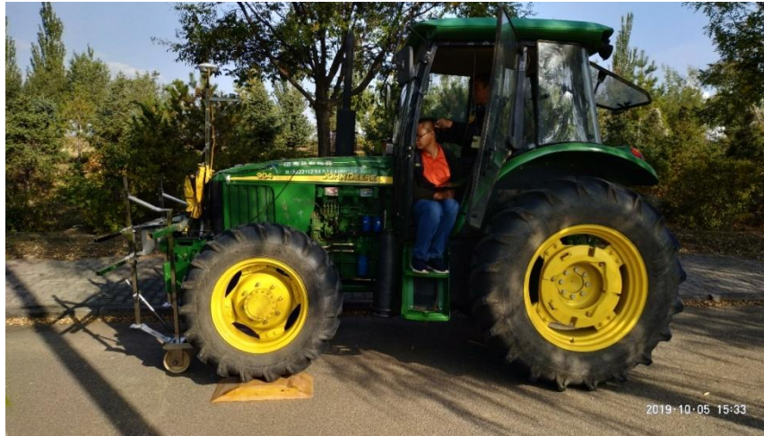
Fig. 5 - Asphalt road profiling validation test
